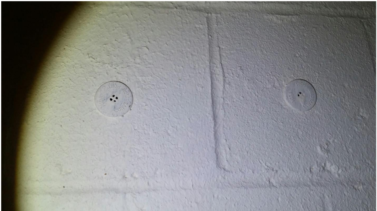
These vents need to be cleaned.
