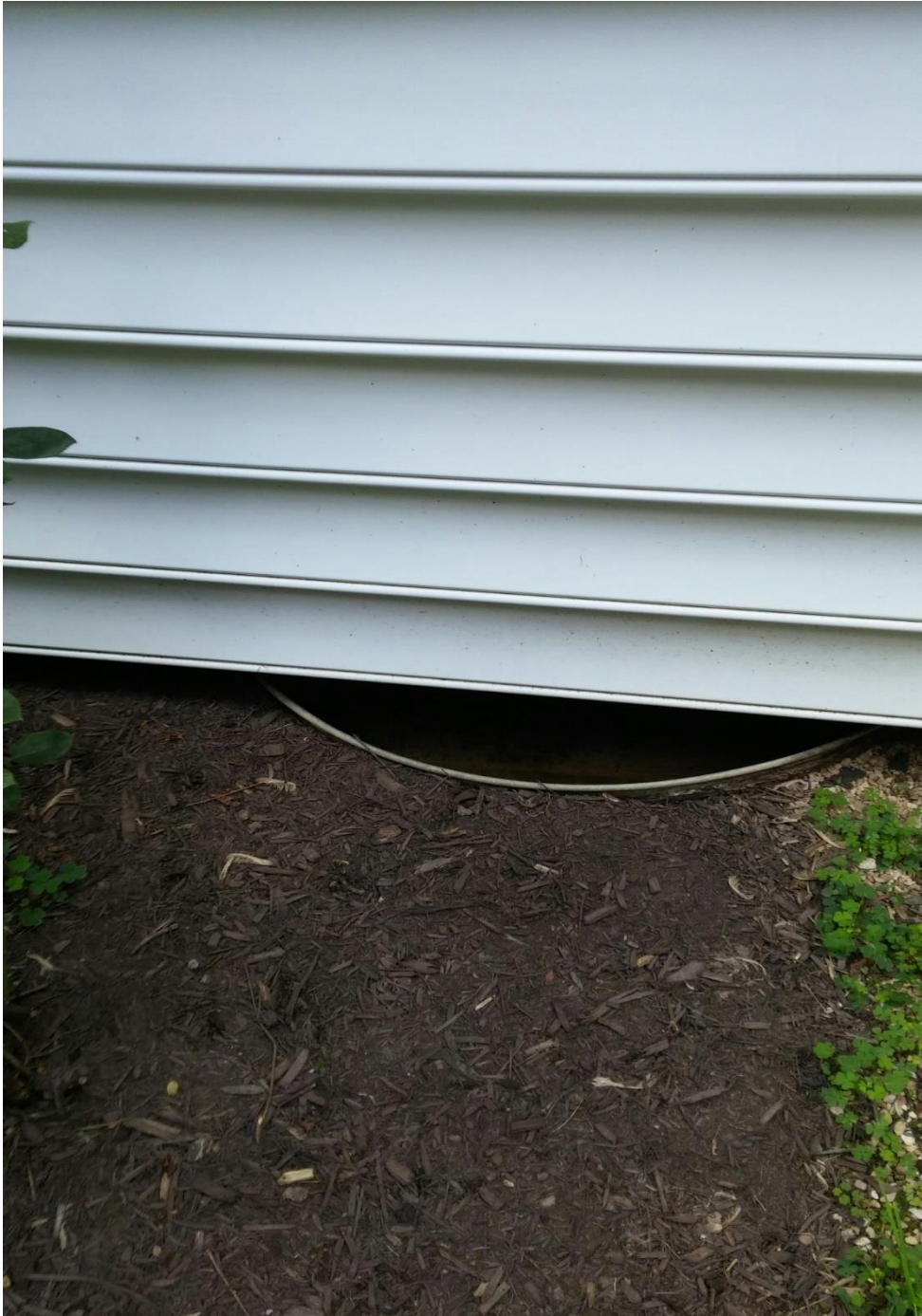
Window well catching siding overflow.
