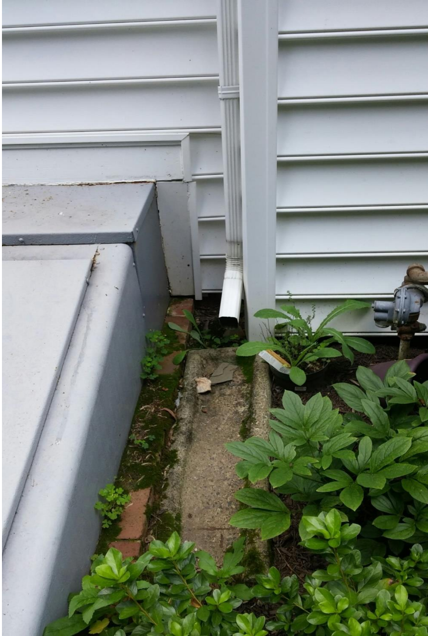
Downspout extension needed here.
